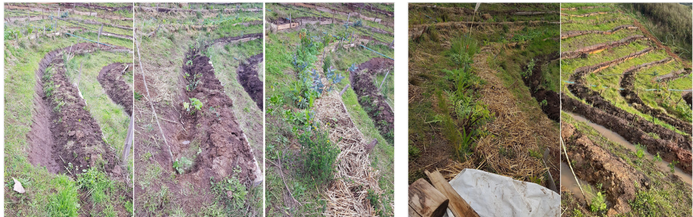
Figure 27. Slope stabilization and plantation using keylines.
