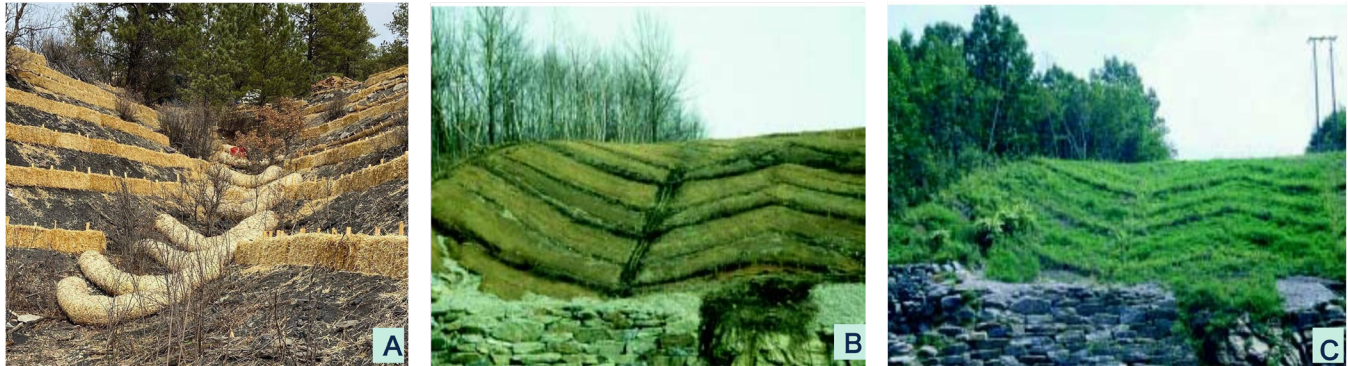
Figure 26. Examples of slope stabilization projects: A- El Ratón Nuevo México; B & C: Robbin Sotir & Associates [Gray & Sotir, 1996].
